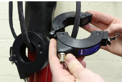
Figure 4: Connecting an RFCT to the earth of cable terminations
