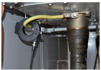
Figure 2 RFCTs installed on the earth conductor of single-core cables.
