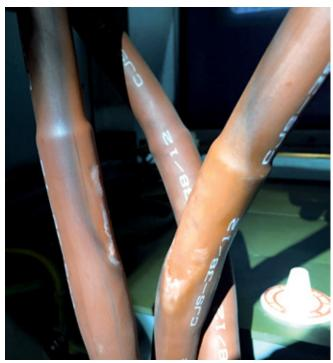
**Figure 1** Partial discharge caused by incorrect installation found on a cable termination using non-intrusive PD 'UltraTEV' instrument
