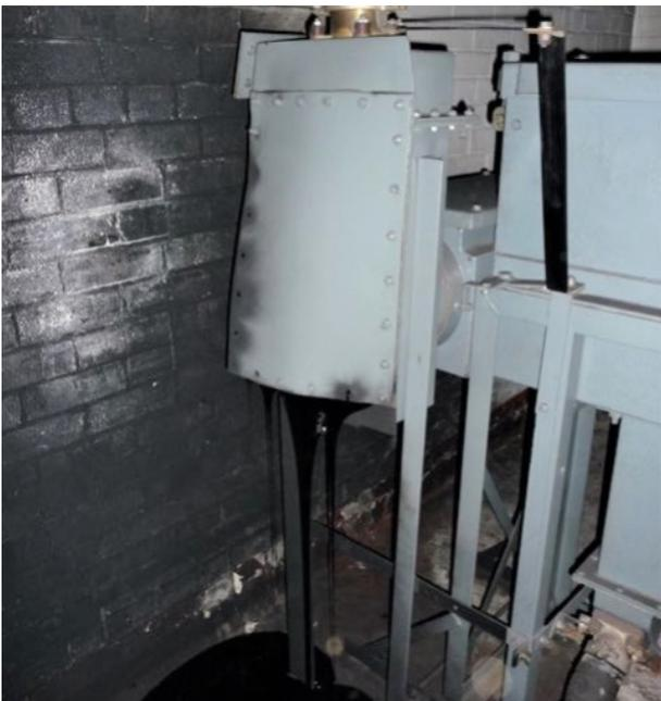
Figure 1 Failed bitumen filled cable box
