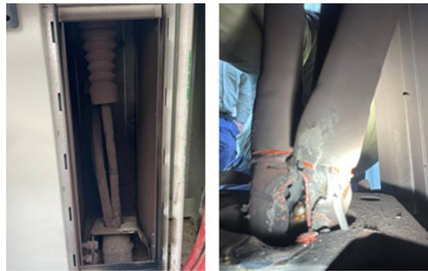
Figure 4 11kV RMU Termination Failure
