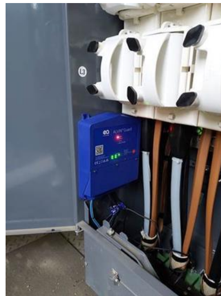
Right: ALVIN® Guard Pre-fault detector in-situ
