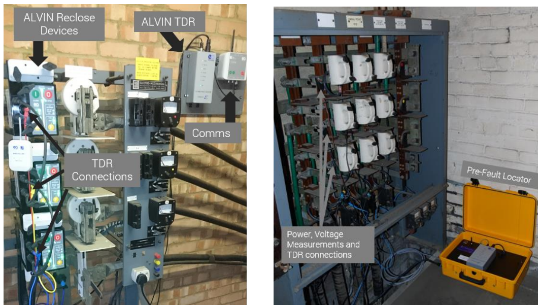
Figure 7 Left: Locate and Manage Equipment Right: Locate Only using Prototype Pre-Fault Locator
