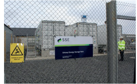
2MW/0.5MWh containerised system, SSEPD
